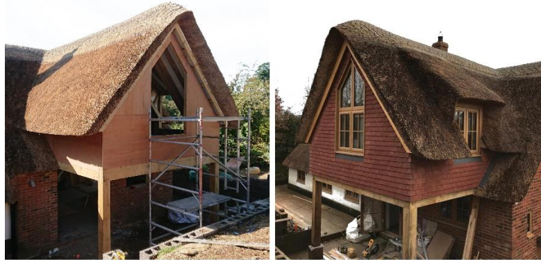
Timber frame extension under construction (left) and completed (right)
